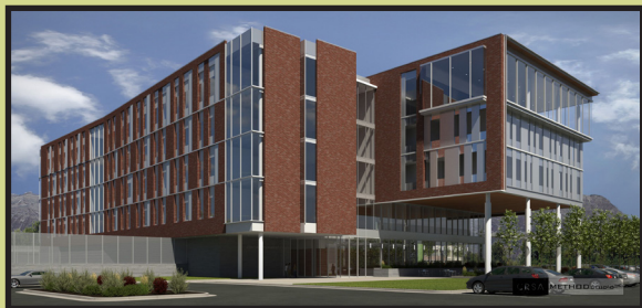
Article adapted from the UVU press release, UVU Officials to Cut Ribbon New Classroom Building ; photo courtesy of UVU Marketing.
