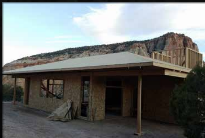
Fig. 8 The new classroom building under construction.
