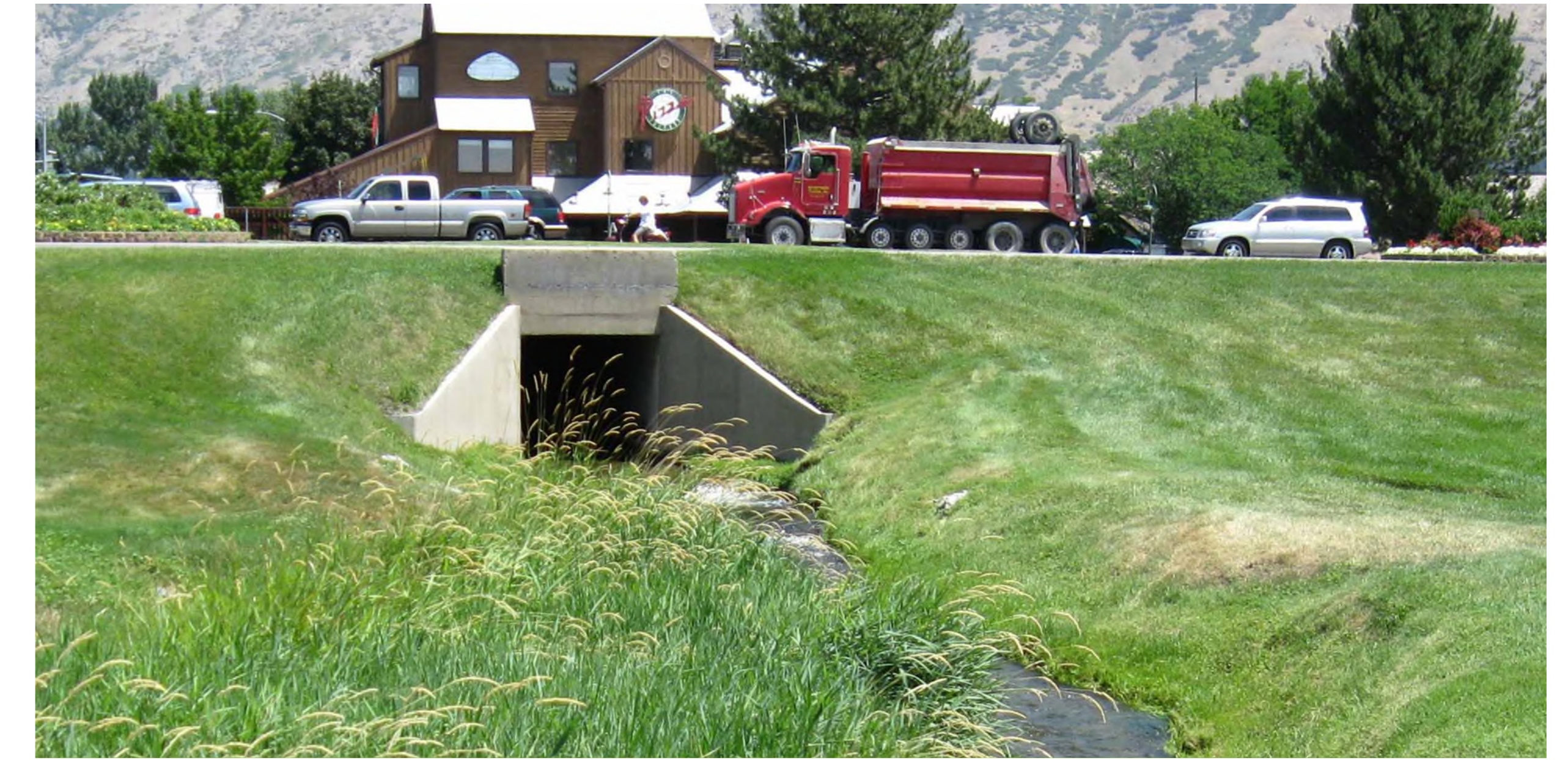
Figure 3. Box Culvert Bridge Further Downstream the Lake Bottom Canal
